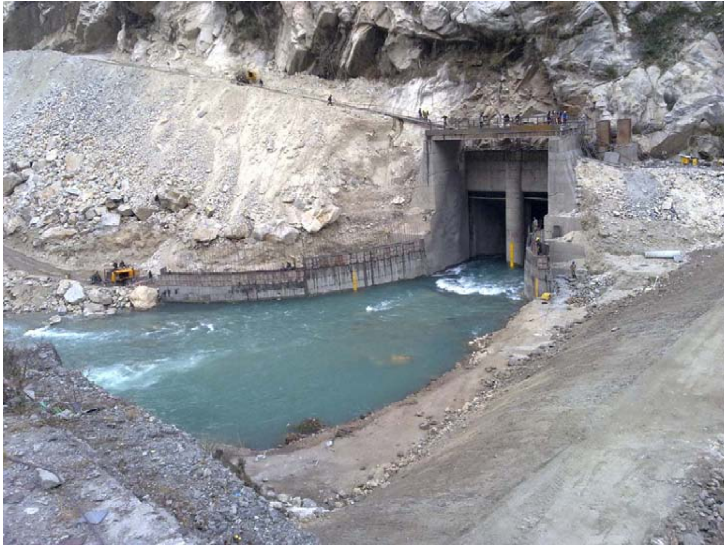
Teesta - 1200MW Run-of-The-River Hydro Power Plant
