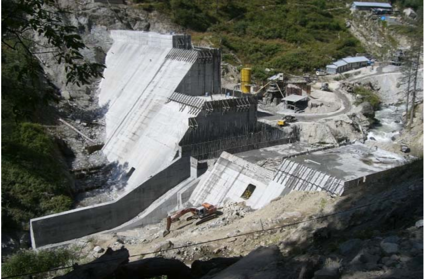
Malana - 100MW Run-of-The-River Hydro Power Plant
