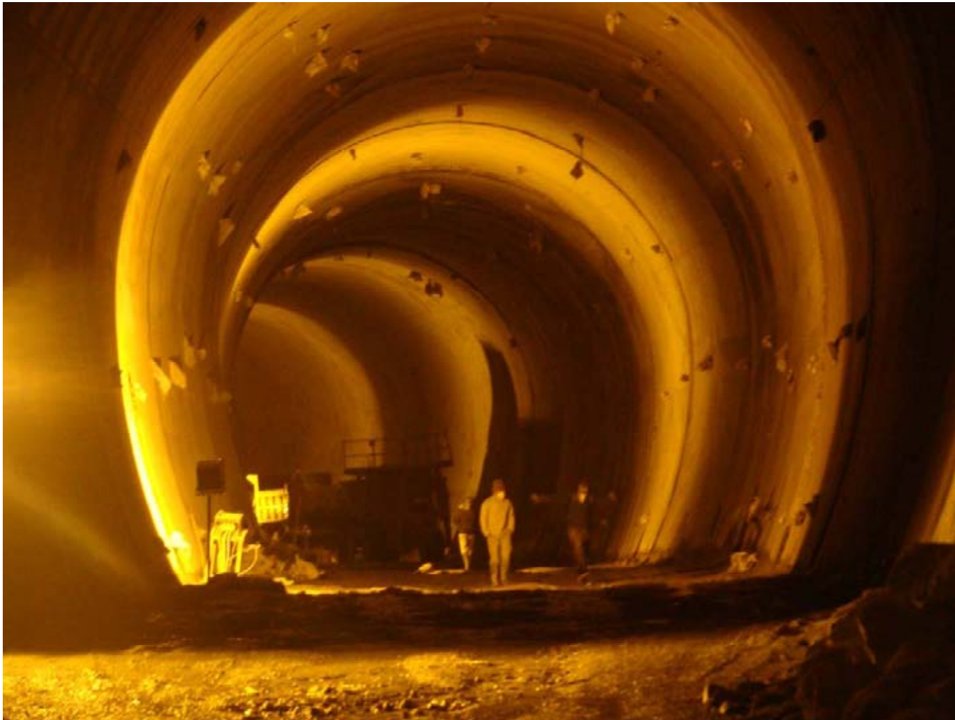
Teesta - 1200MW Run-of-The-River Hydro Power Plant
